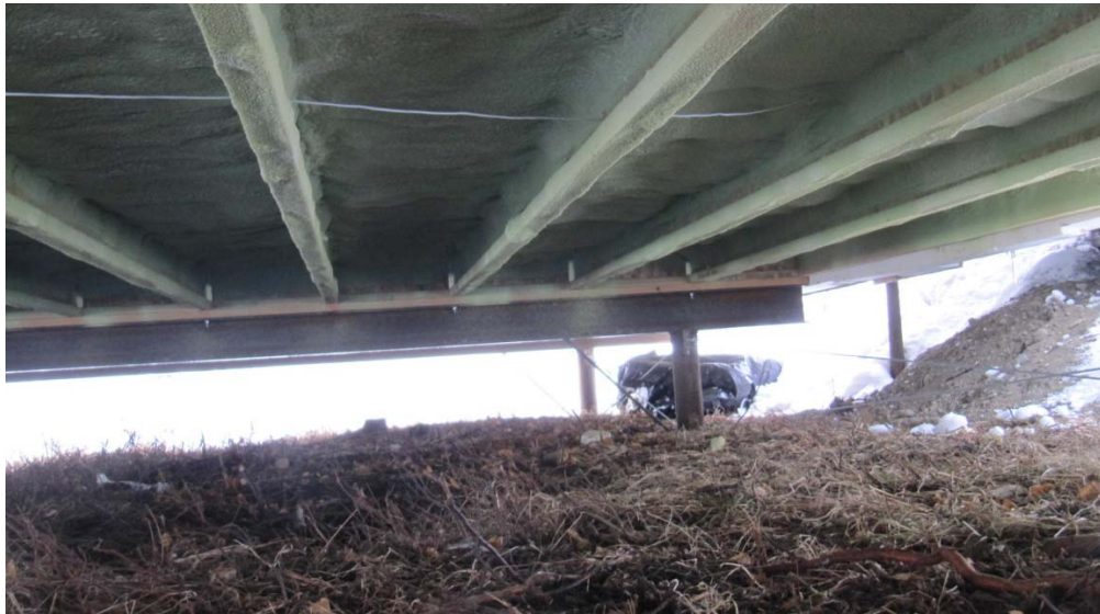
Figure 50. Willow House: Founded on piles with an open crawl space below.
