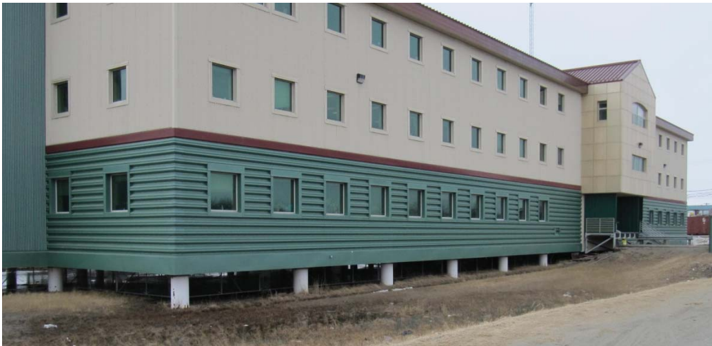
Figure 5. Example: Open ventilated crawl space to protect permafrost under a heated building.
